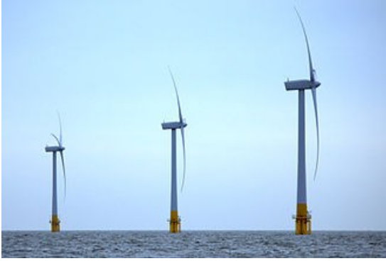
Figure 6: Offshore Horizontal Axis Wind Turbines (HAWTs) at Scroby Sands Wind Farm, UK
